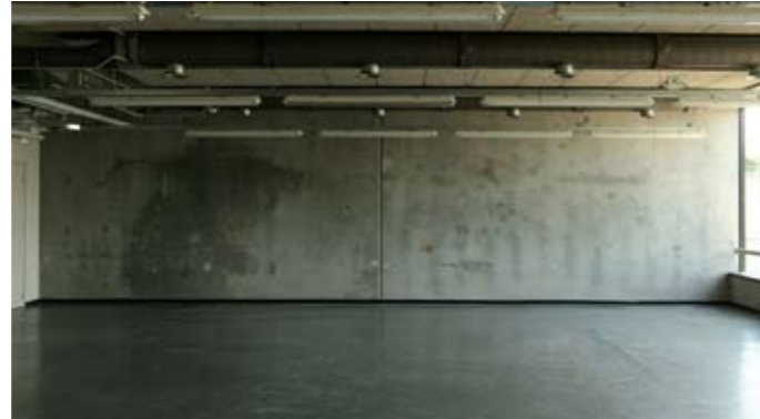
why bridges won't fall , overview photo
